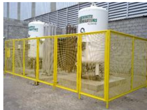
Figure 4: After Cleaner Production: Gas Station
