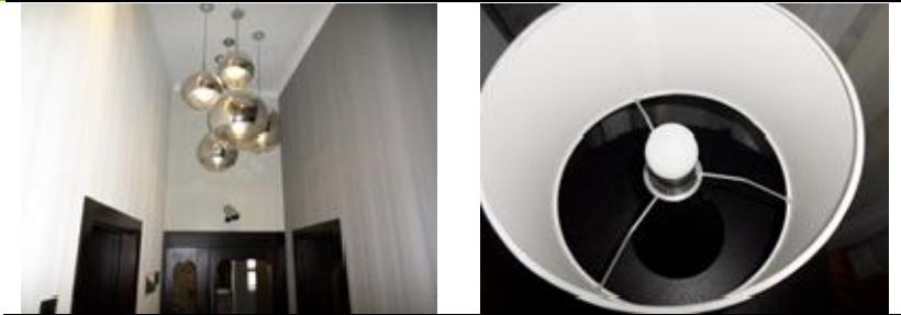
Figure 2: Led lights in place
