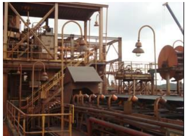
Figure 3: After Cleaner Production : With a behavioral change, it uses the illumination system only when necessary
