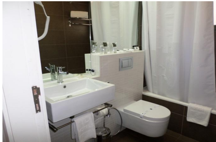
Figure 6: Dual flush tanks and water flow regulators in taps and shower caps
